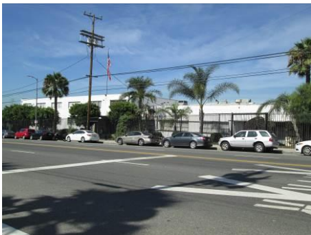
Address: 15001 S. Figueroa Street Date: 1954 Name: Burg Tool Manufacturing Company
