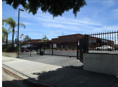
Address: 18349-18355 S. Figueroa Street Date: 1956 Name: Steambitters, Welders, and Refrigeration Fitters Union Hall
