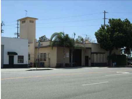
Address: 18030 S. Vermont Avenue Date: 1941 Name: Fire Station #79
