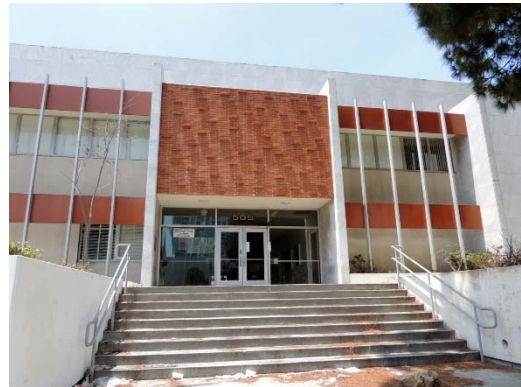
Address: 505 s. Centre Street Name: San Pedro County Building Date: 1968
