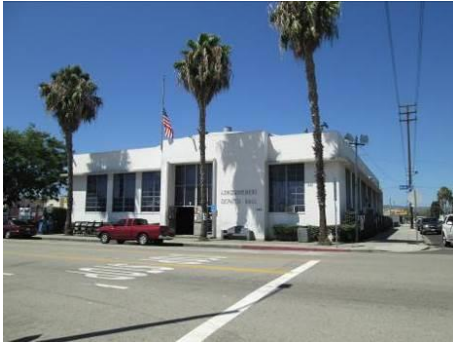
Address: 122 E. D Street Date: 1947 Name: Longshoremen's Dispatch Hall
