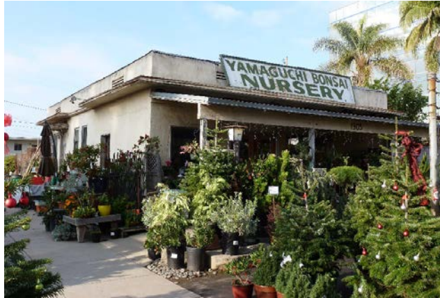
1903 S. Sawtelle Boulevard, 1934 Yamaguchi Bonsai Nursery was established at this site in 1949 (SurveyLA)
